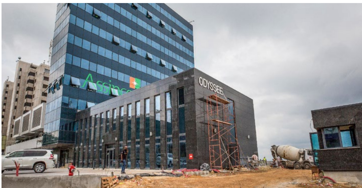
"Odyssée", the new head office, under construction.
